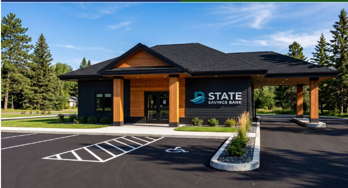
State Savings Bank Garden Branch
